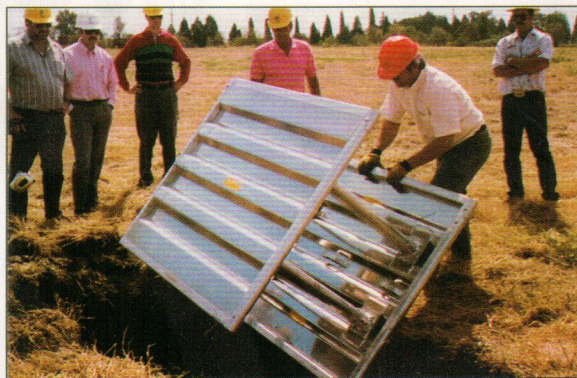
Installing in Trench Becomes a One-Man Job
