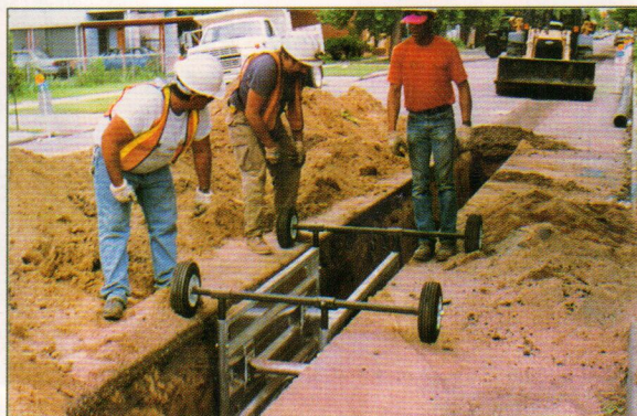
Wheel Kit Speeds Work and Increases Pipe Clearance
